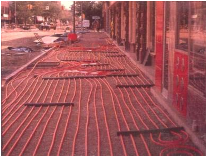
Klamath Falls snow melting system
